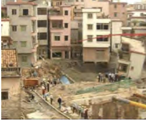
**Figure 2** Results of a tunnel collapse in a residential area showing the possibly very large extent.
